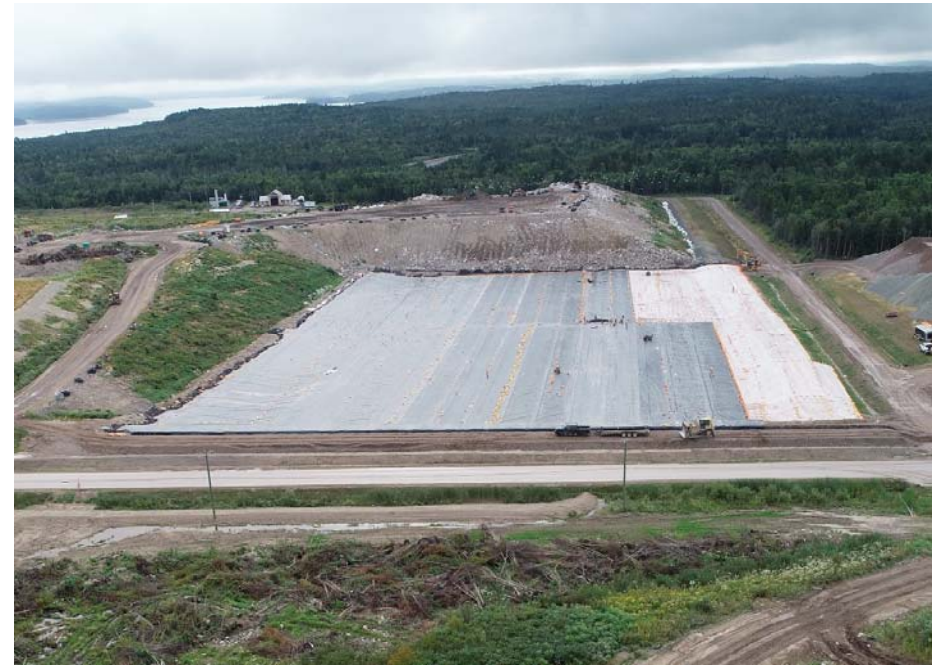
Crane Mountain Landfill Cell 9 Construction (2022)
